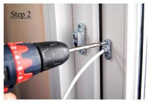
Position the restrictor unit (A) on the opening frame. Directly screw provided self drilling screws (E) with a crosshead screwdriver. Alternatively pilot holes can be pre-drill with a 3 mm drill bit for ease of installation ( although not essential ).
