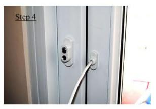
Clip plastic cover (B) in to position over the lock unit (C).
