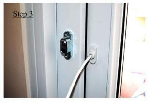
Clip plastic cover in to position over the restrictor unit (A). Once clipped, children can not remove plastic covers easly and reach screws.
