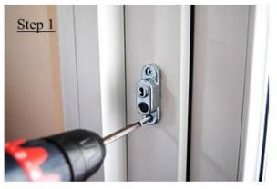
Position the lock unit (C) on the fixed frame. Directly screw provided self drilling screws (E) with a crosshead screwdriver. Alternatively pilot holes can be pre-drill with a 3 mm drill bit for ease of installation ( although not essential ).
